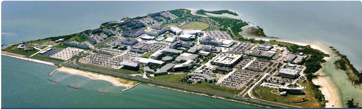
Aerial Image of Texas A&M - Corpus Christi
