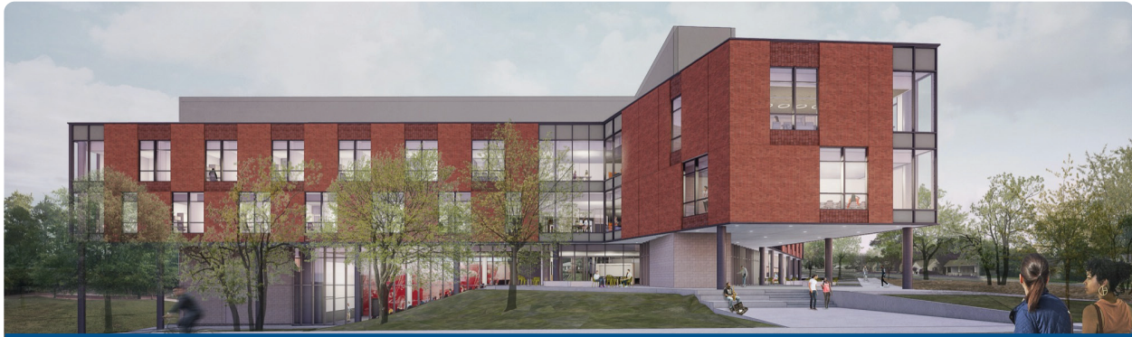
North Carolina School of Business, Computer Information Systems Department
