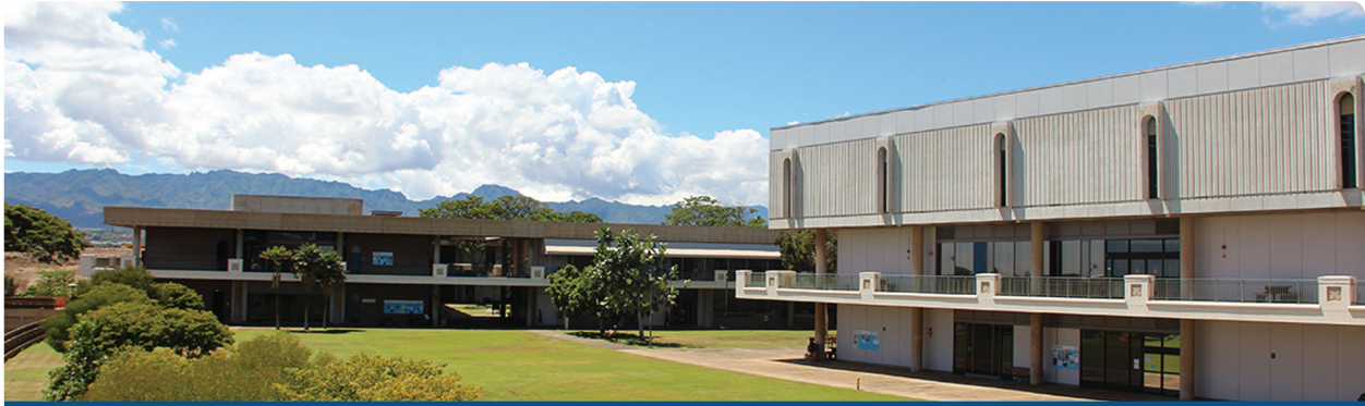
Pu'uoloa Campus at Leeward CC
