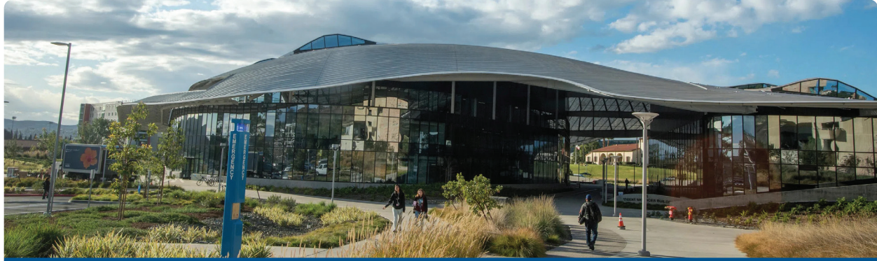
CPP Student Services Building
