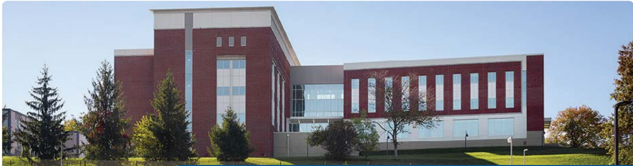
The Advanced Engineering Research (AER) building houses the Lane Department of Computer Science & Electrical Engineering and many of WVU's Cyber programs
